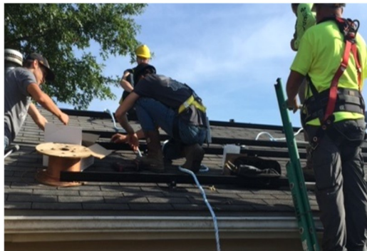
Electricity Installing Solar Panels
